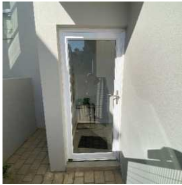
Typical unit doors
