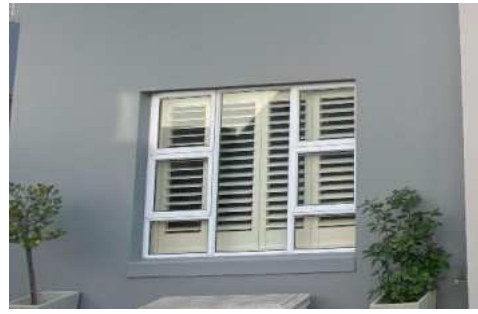
Typical aluminium windows
